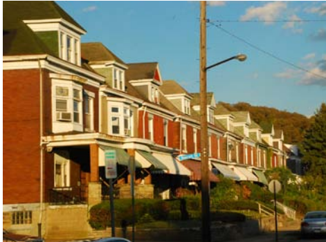
Renovation of Existing Housing
