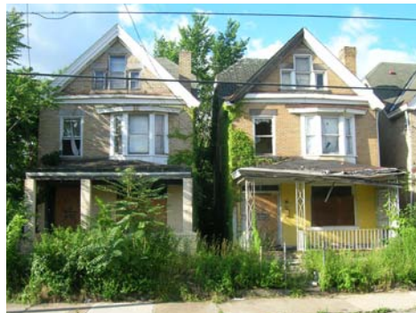
Vacant Houses on Tioga Street
